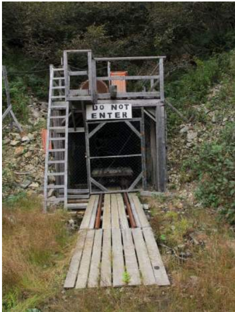
Adit entrance showing ventilation fan
